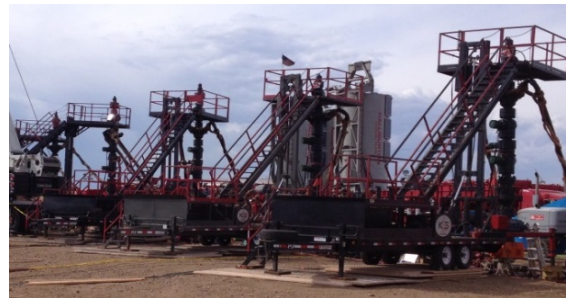
Five (5) well pad with combination of Guardian's Stage Isolation Tool and Zipper Manifold.
